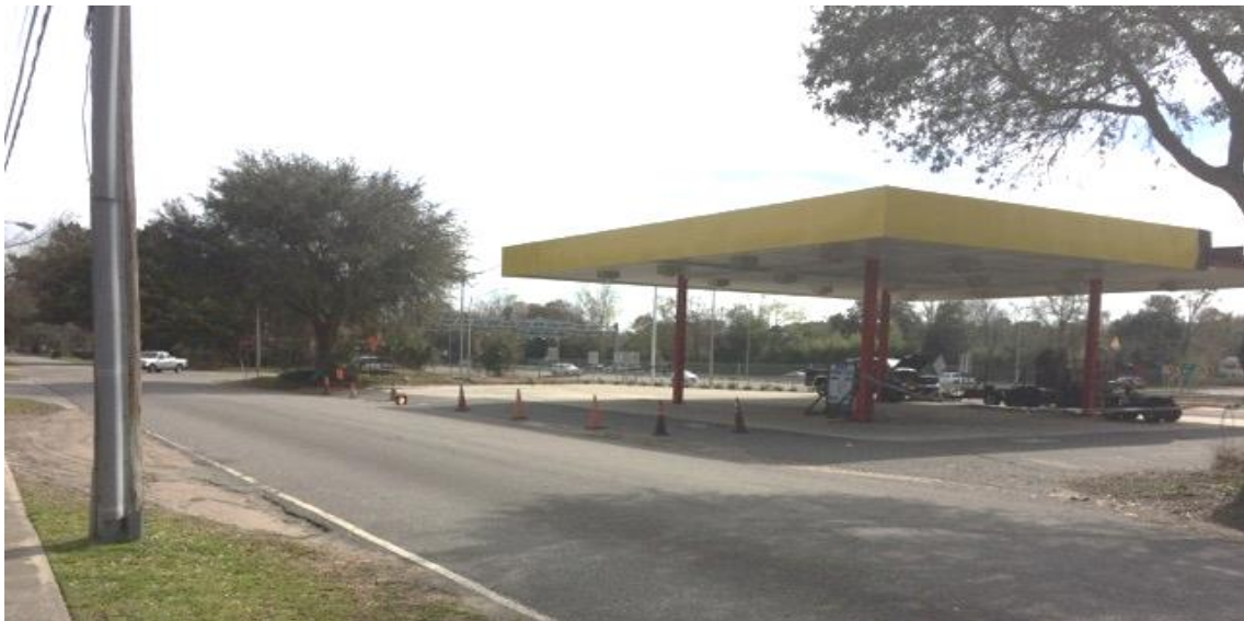
Facing southeast at the subject site from the Flash Foods store across Devoe St
